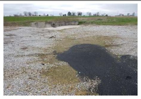
Storm water retention basin with sluice gate. Note black sand fill.
